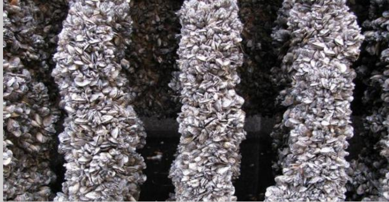
Dam Intake Tower
